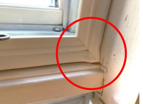
Alpina's Storm Snaps' attractive, finely mitered corners with commercial quality EPDM press fit rubber trim make for fully sealed, highly attractive corners.
